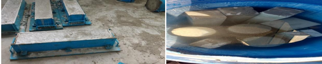
Fig (j): Casting and Curing of Beam moulds
